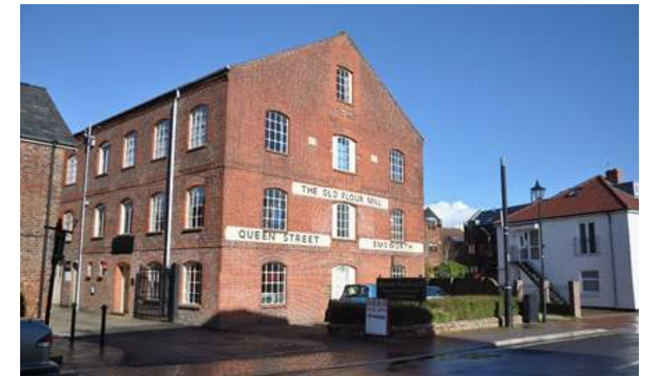
FLOUR MILL, QUEEN STREET
