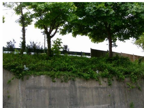
Plate 4: Retaining wall with scrub and trees
