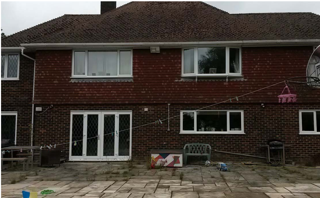
Photograph No. 02 - View of the southern aspect of the existing building on site.
