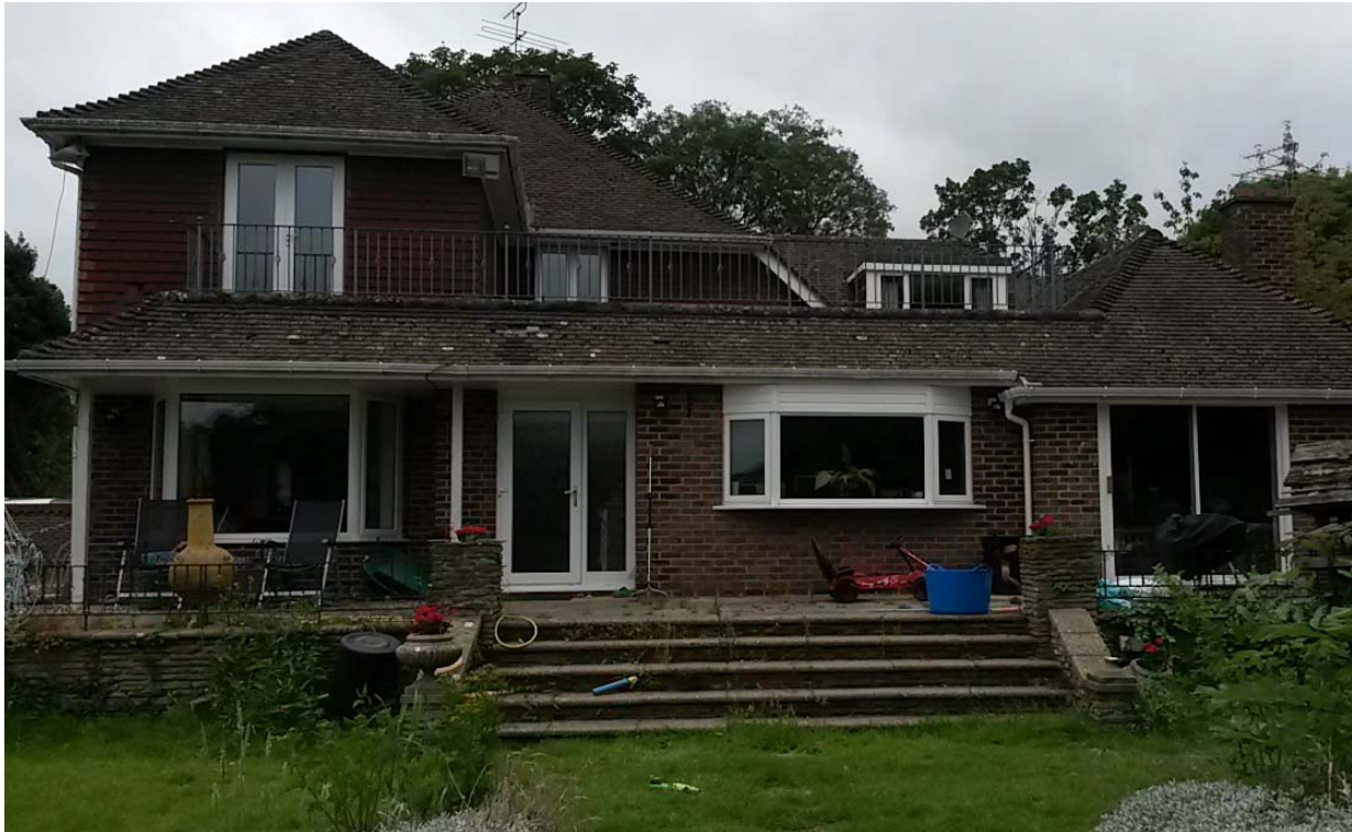
Photograph No. 03 - View of the eastern aspect of the existing building on site.
