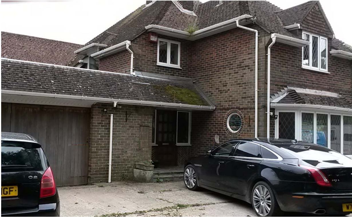
Photograph No. 01 - View of the western aspect of the existing building on site.
