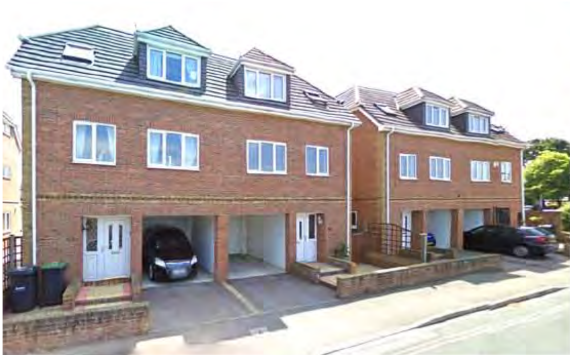
5. EXISTING 2.5 STOREY TOWN HOUSES ON ST MARY’S ROAD, ADJACENT TO THE NORTH WEST SITE BOUNDARY
