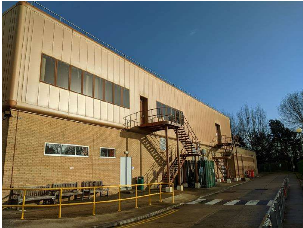
Photo 3 – Buildings to the east are largely brick but still offer negligible bat roost potential.
