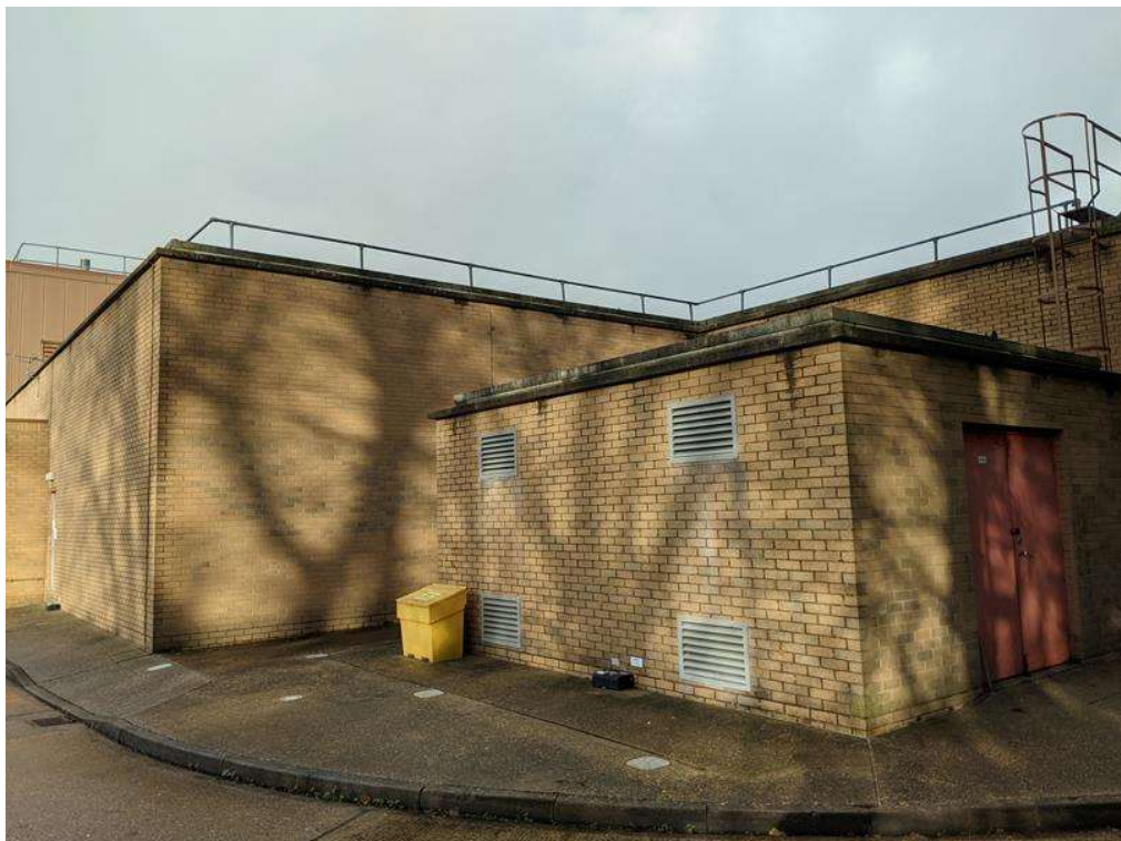
Photo 2 – Buildings to the east are largely brick but still offer negligible bat roost potential.
