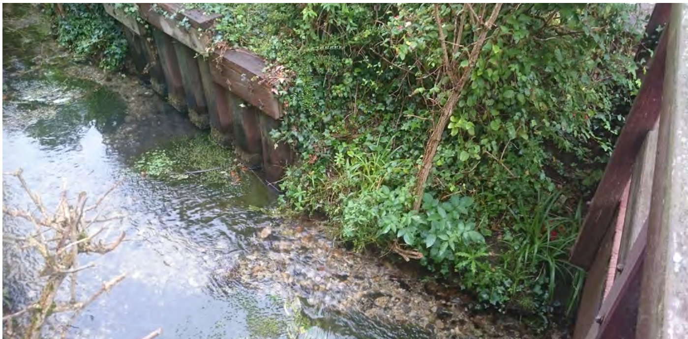
Photograph No. 5 - One burrow entrance, located at TN01, c. 2.00 metres downstream of bridge.
