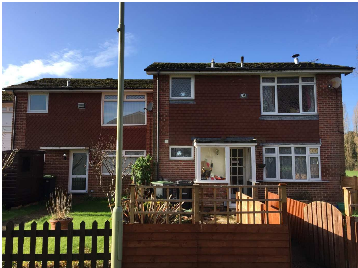
PIC 01_Front view of the existing end terrace No 11 dwelling and the adjoining property at No 10
