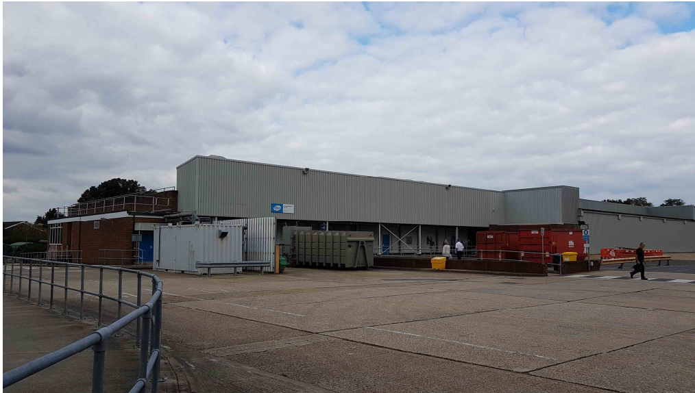
Photograph 5 View of Service Yard at Rear of Building V
