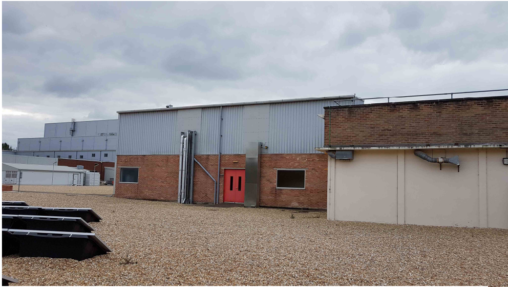
Photograph 8 North Elevation of Building V
