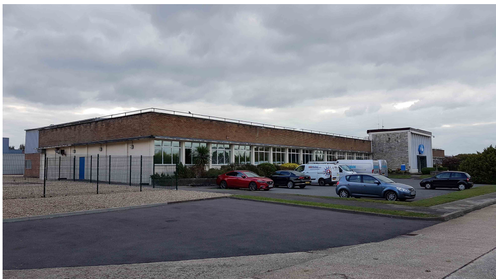
Photograph 1 View of Western (New Lane) Elevation From North West Corner of Site
