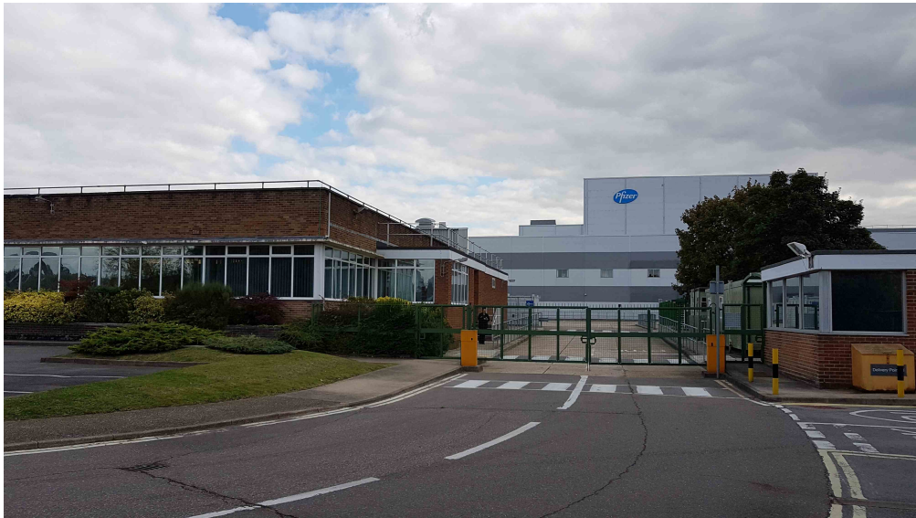
Photograph 3 View of South Western Corner from Access Road
