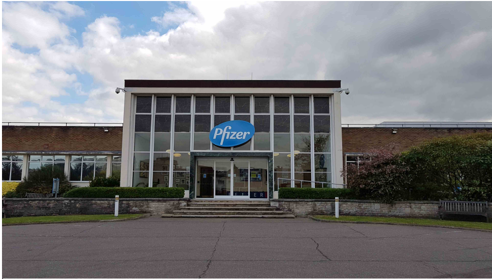
Photograph 2 View of Main Entrance Looking from New Lane
