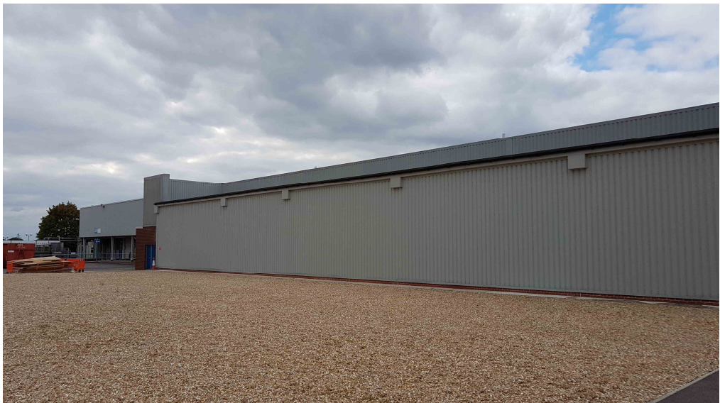
Photograph 6 View Looking Towards Rear of Building V
