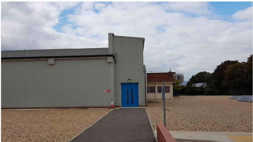
Photograph 7 View Looking Towards Rear of Building V at North Eastern Corner
