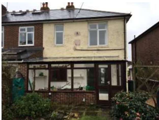
Fig 2, 14 Bath Road, rear extension.
