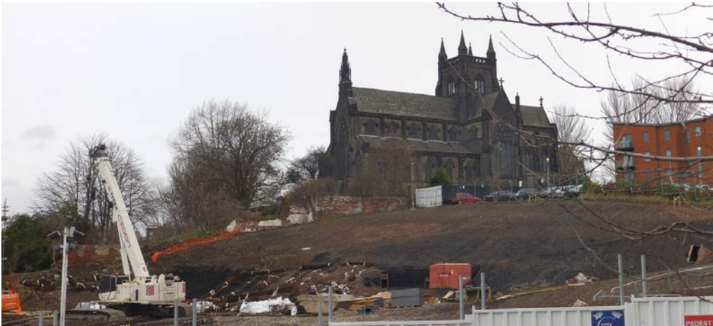
Aire – East Street Leeds under construction
