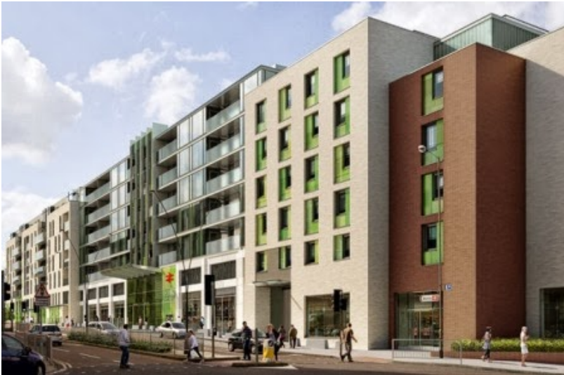
Redevelopment of Epsom Railway station (built)
