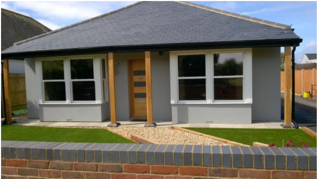
003 - The Retreat now after renovations complete
