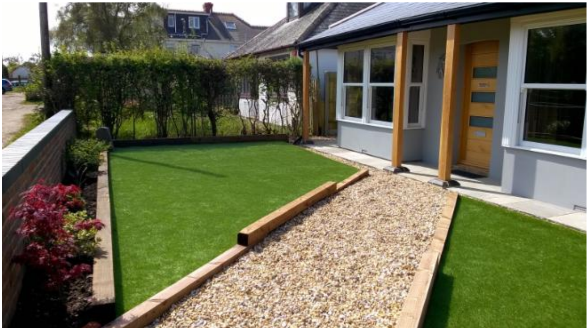
004 - The Retreat now after renovations complete
