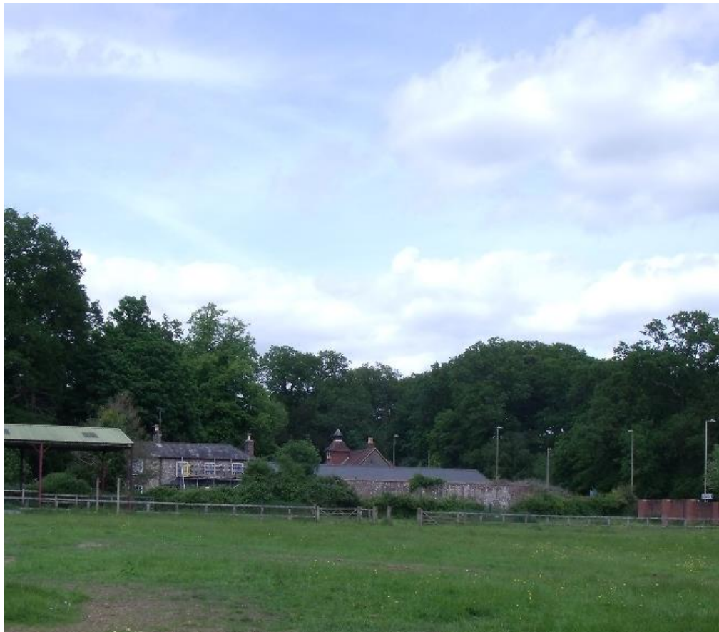
View of Stable Cottage and Stable Block from Storey Gardens
