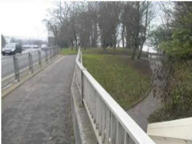
Photo 4.1: Access ramp to Maurepas Way underpass
