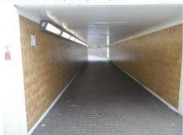
Photo 4.2: Maurepas Way underpass
