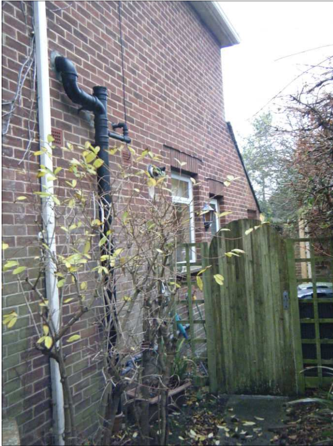
Side view (service) side of house.
