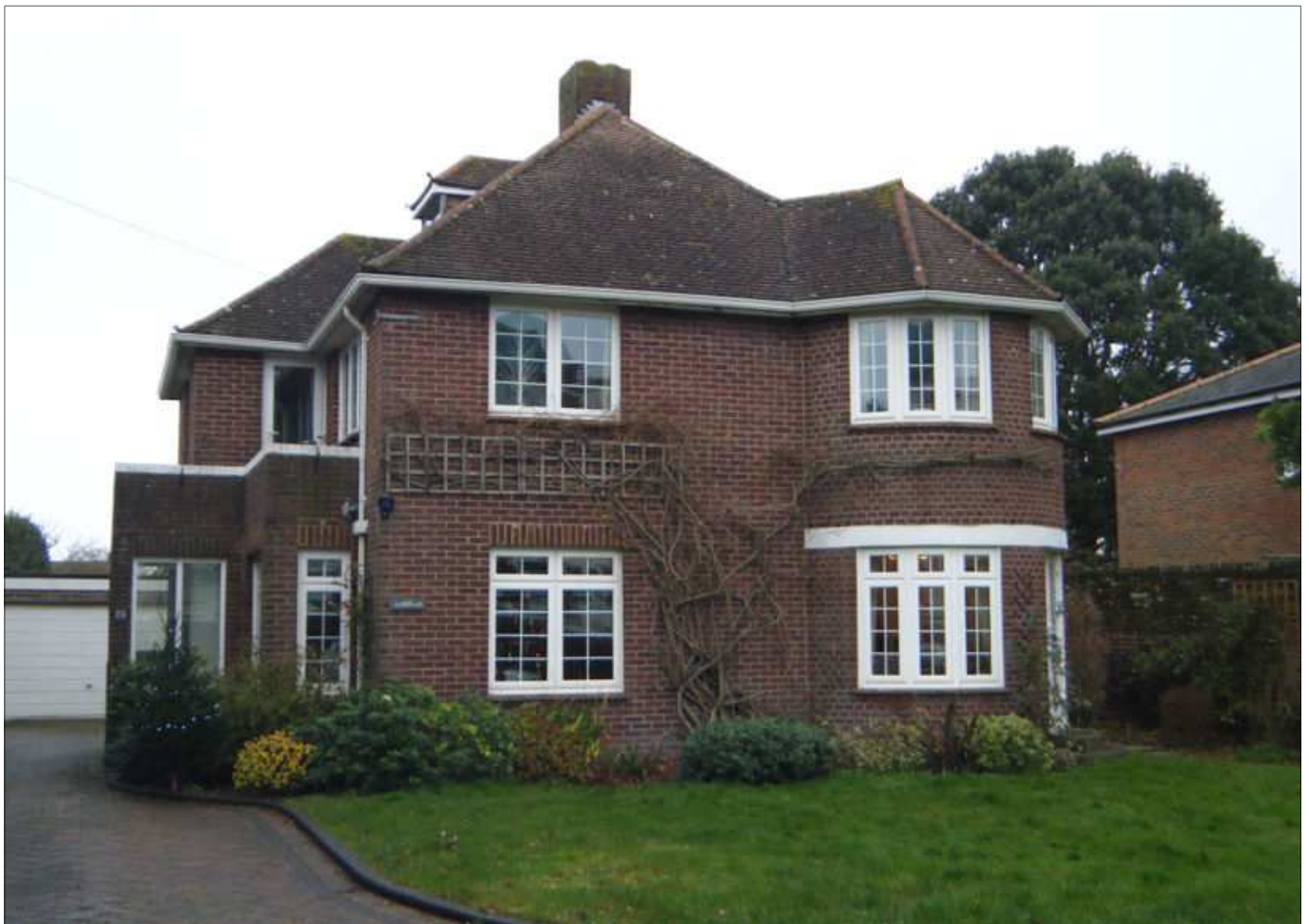
Front view of East Acre, note red brick and sandstone detailing.
