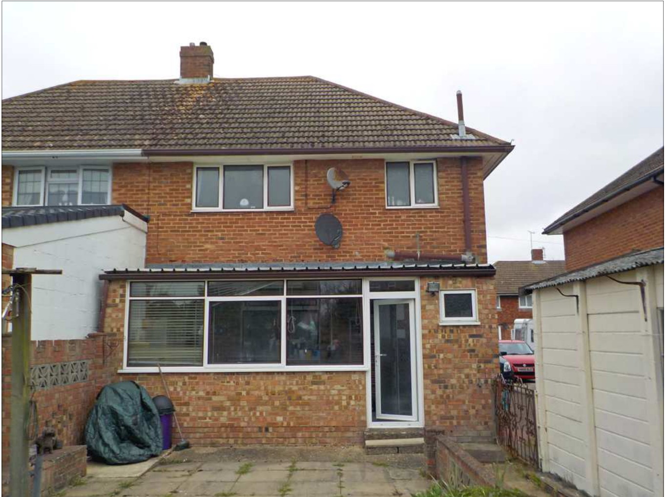
Rear of No. 35 Roman Way - shows existing rear extension
