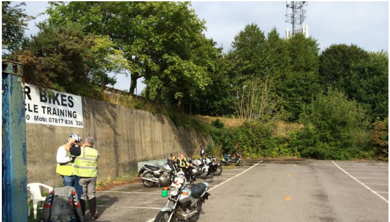
Fig 8 Rear retaining wall.
