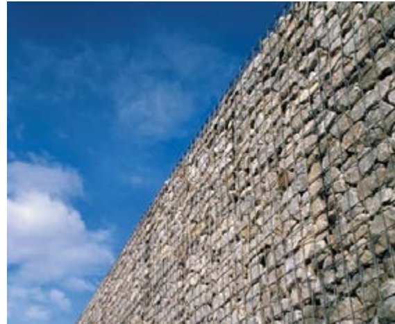
Gabion retaining walls provide aesthetic interest and blur the line between landscaped and natural
