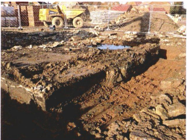
Photograph showing tank base prior to removal
