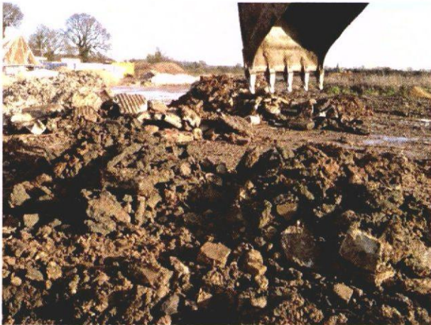
Photograph showing the waste materials from the excavation works
