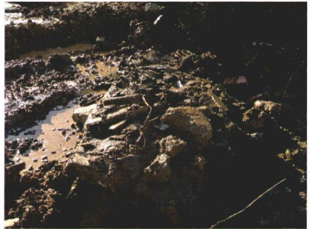
Photograph showing presence of asbestos containing materials within the concrete slab of the boiler house
