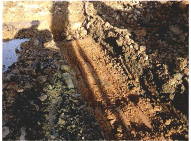
Photograph showing the eastern side of the tank base excavation
