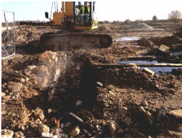
Photograph showing the removal of the base and short section of duct
