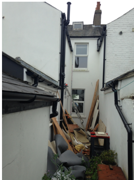
Rear Area (looking from rear gate)
