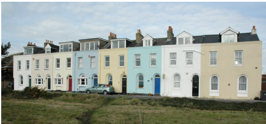
South Facade (subject property white house at right)
