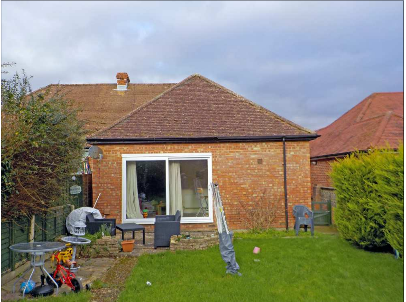
Rear of No. 48 Bushy Mead
