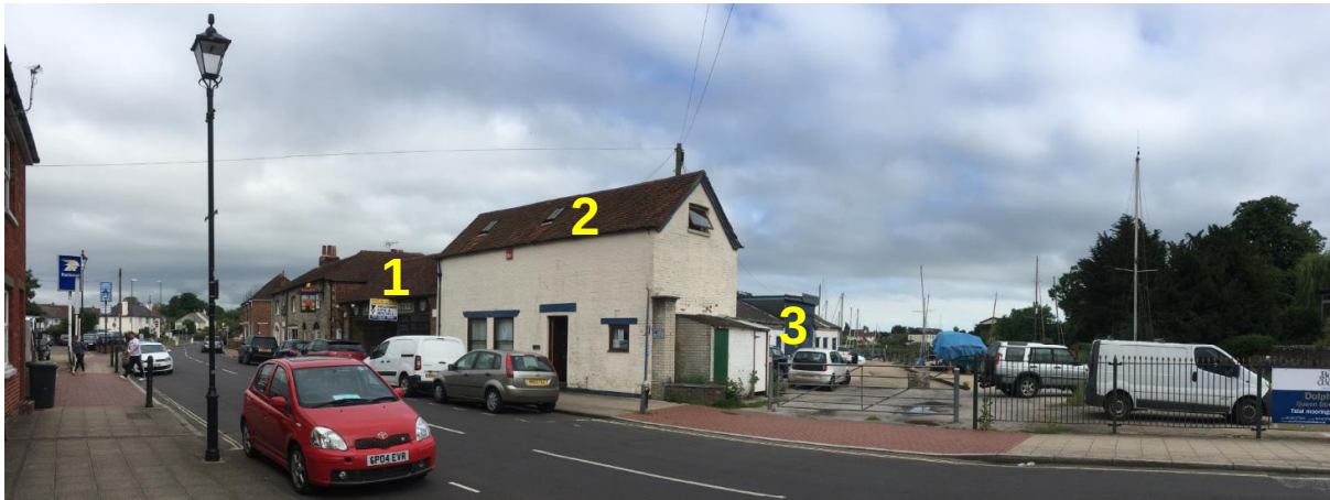
Above: View from North-West along Queen Street towards the Site
