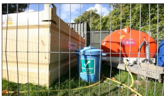
Photo 46: Where fuel or other chemical are stored on site, it is now standard practice to have emergency spillage kits available to restrict the environmental impact of accidents.
