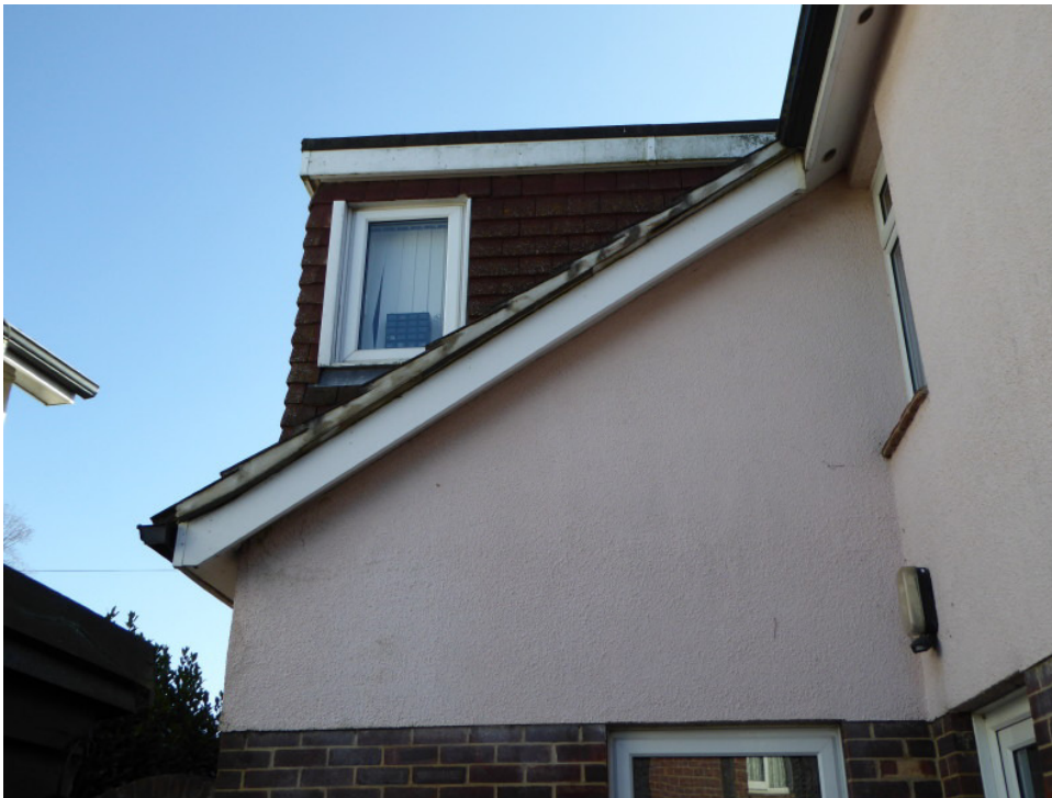
No 29 existing dormer viewed from rear
