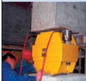
Adjusting a spring unit – Shanghai, China
