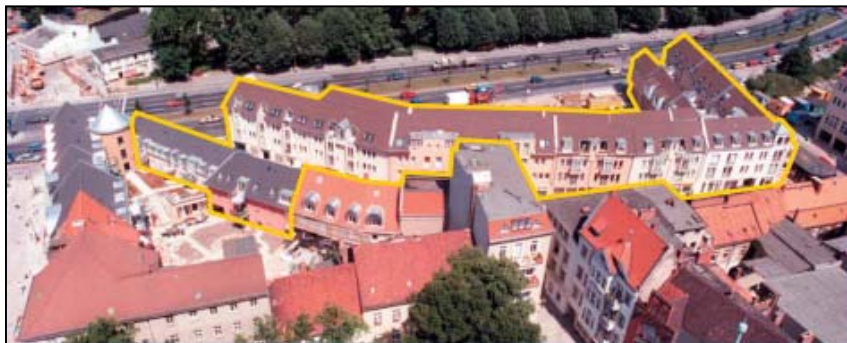
Complex of buildings above an underground line on 5 Hz spring units – Berlin, Germany
