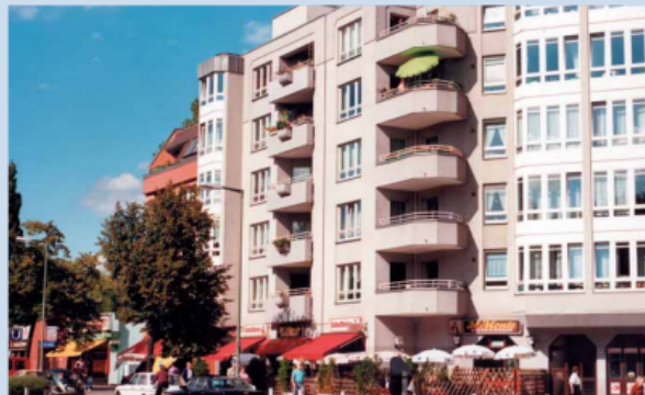
The worldwide first residential building spring supported for vibration isolation, 4 Hz – Berlin, Germany 1986
