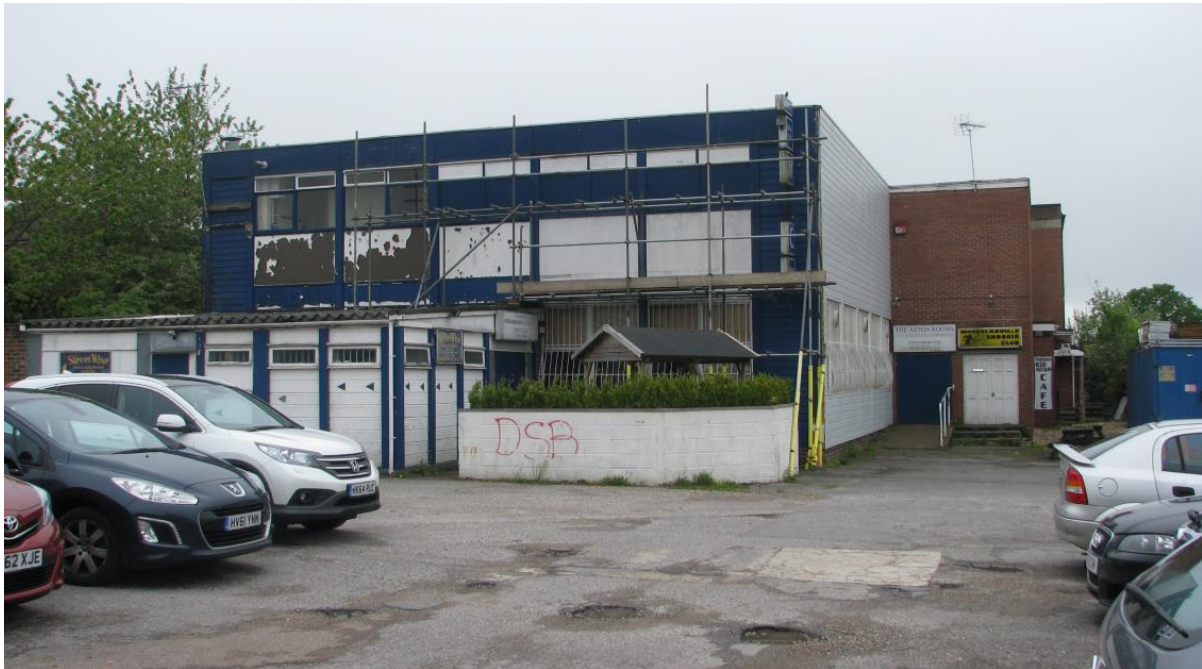
Above: North-East Elevation of Existing Building
