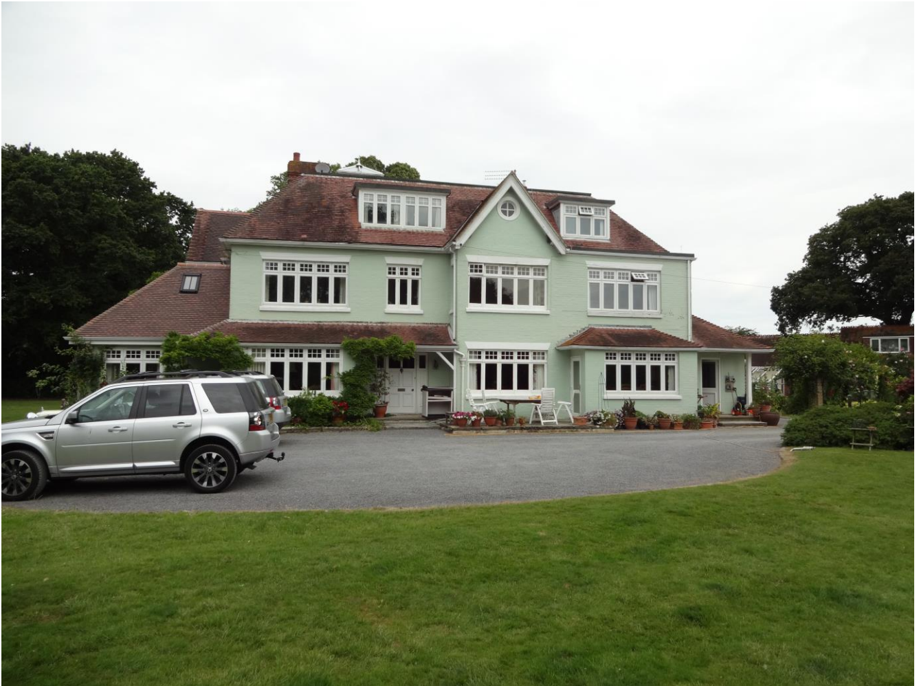
South-East Elevation of Littlemead House
