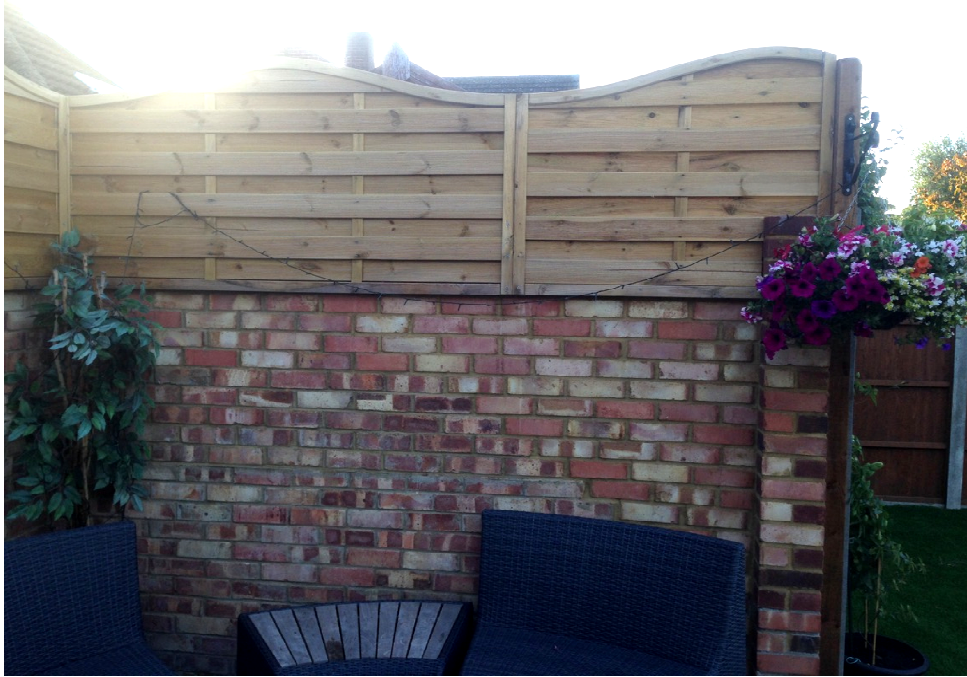
View of eastern boundary wall facing garden of no. 5 Berkeley Square.
