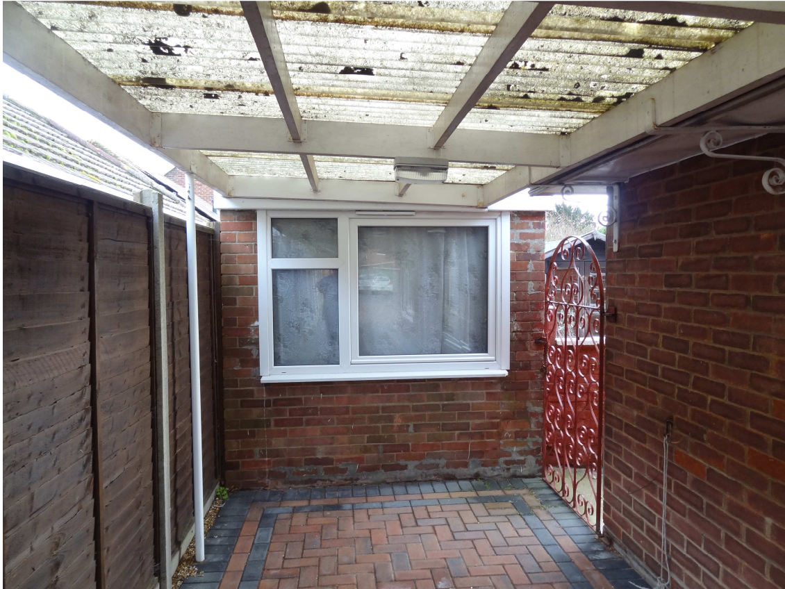
Outbuilding prior to demolition - Note height of building above adjacent boundary fence.
