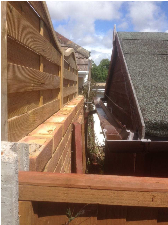
View looking behind eastern fence showing existing shed in garden of No. 5.
