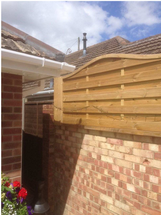
New northern boundary wall & fence facing no. 7 Berkeley Square.
