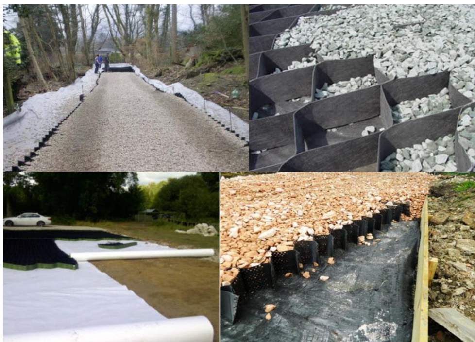
Figure 4. Photographs illustrating cellular confinement system used to form an above-ground no-dig driveway.
