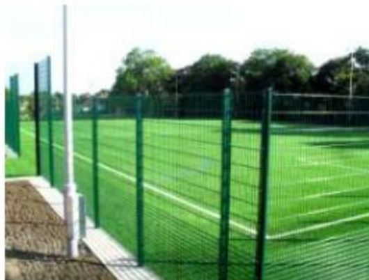
Example of ball-stop fencing
