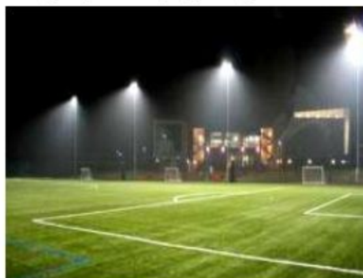
Example of floodlighting
