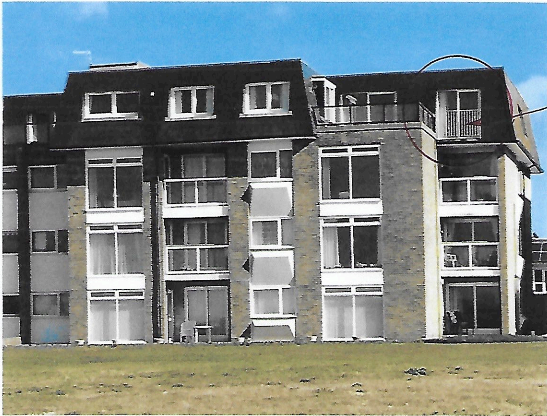
South elevation of 13 Silhouette Court showing full height window
