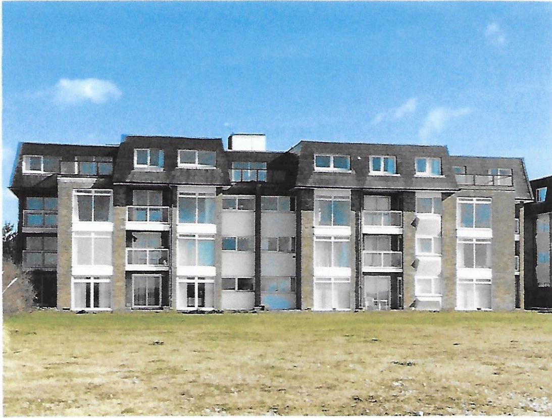
South elevation of Silhouette Court
