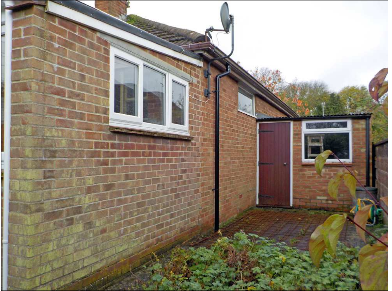
Side of 71 Privett Road showing rear of garage
