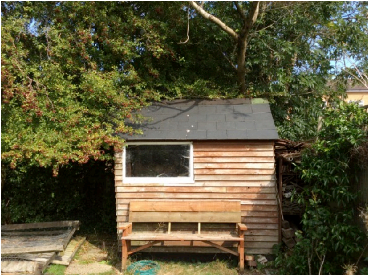
Figure 3 – Wooden shed with bitumen sheet on top ridge.
