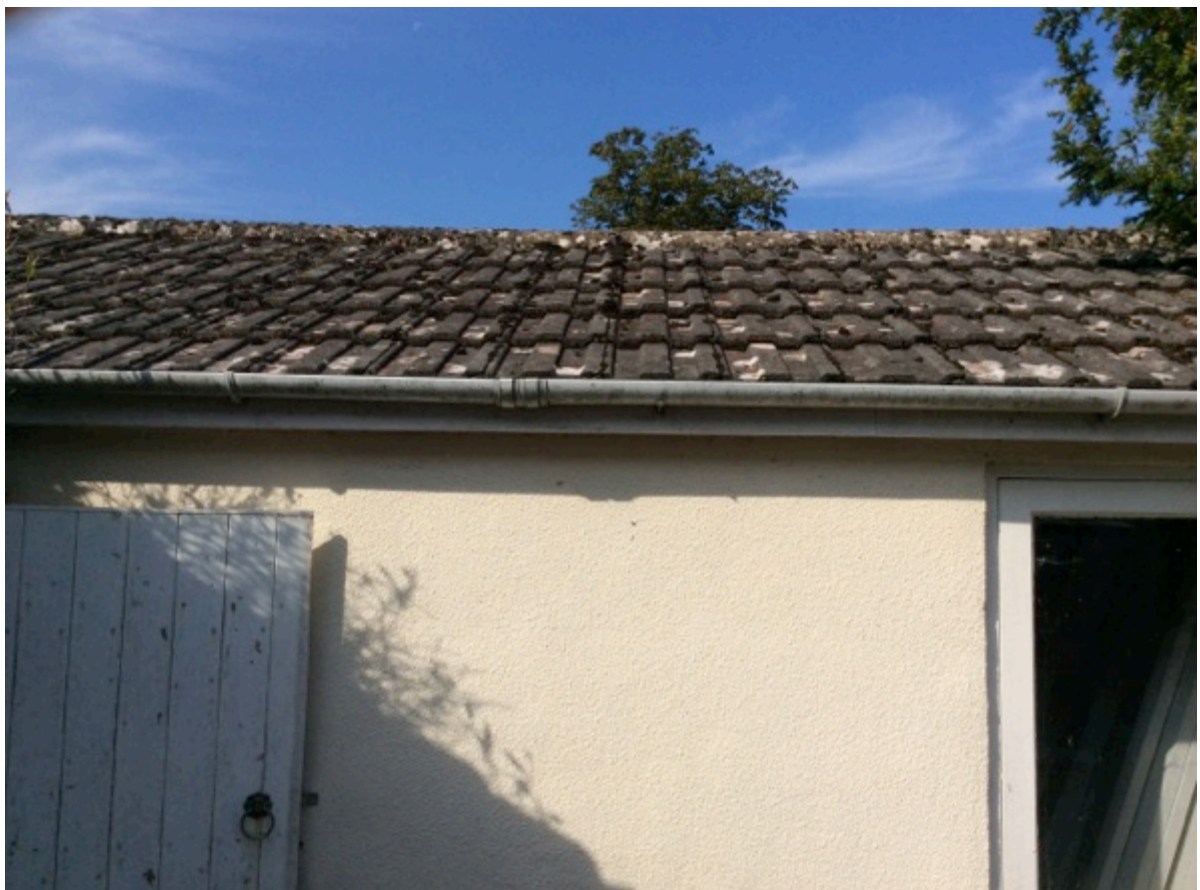
Figure 2 –The roof of the garage with interlocking concrete tiles.
