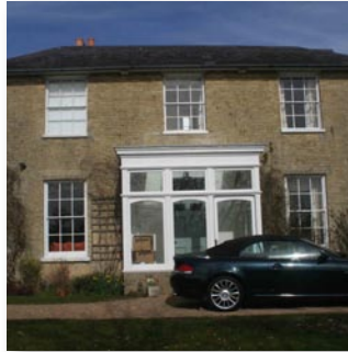
Main Entrance East Leigh House
