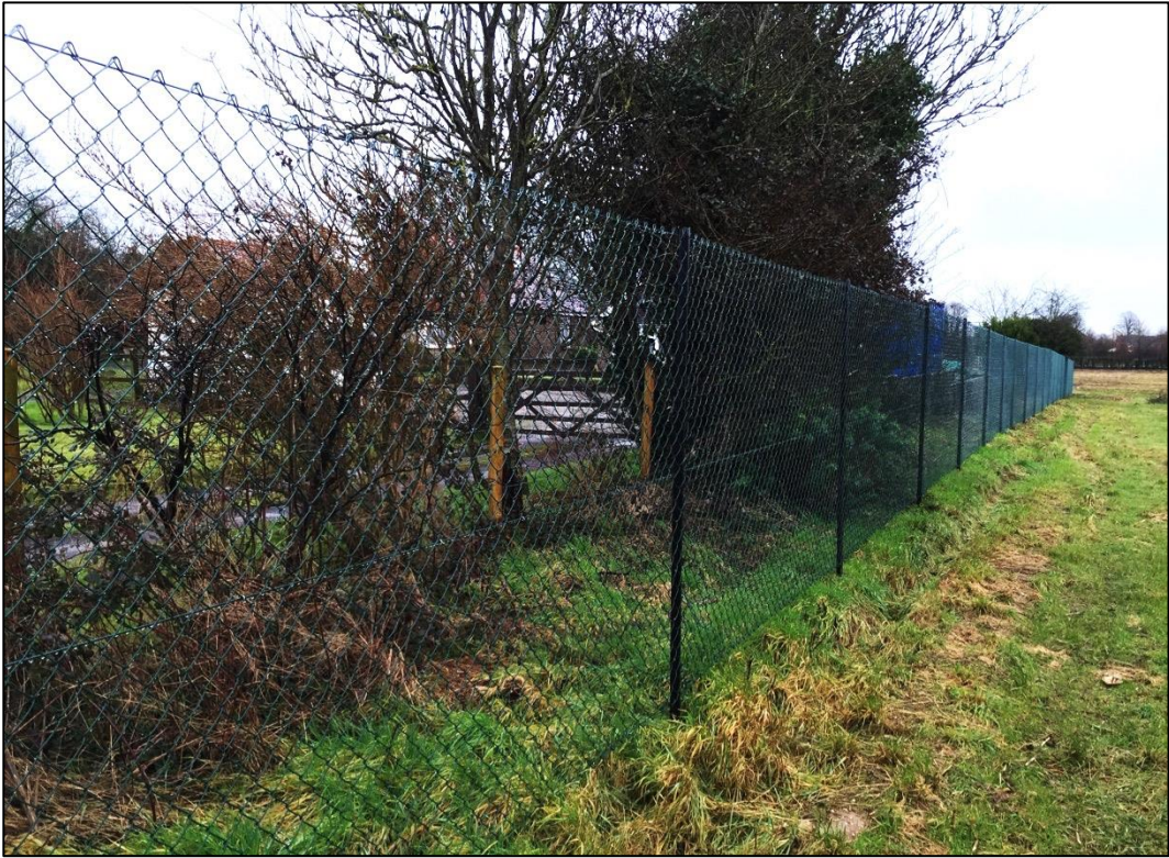
Chain-link on angle-iron uprights
