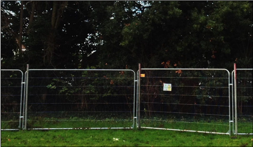
Weld-mesh panels on scaffold uprights
