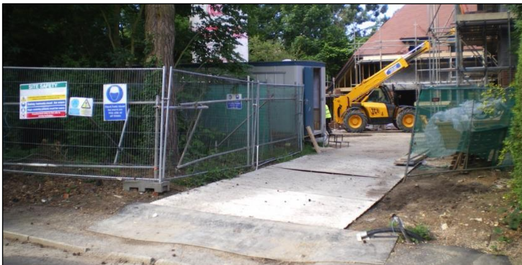
Vehicular ground protection trackway
