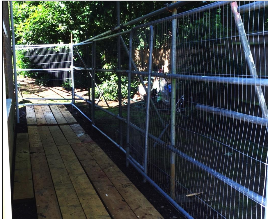
Scaffold board pedestrian ground protection
