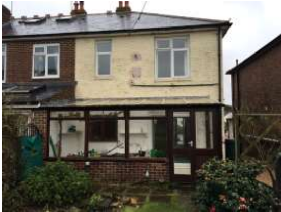
Fig 2, 14 Bath Road, rear elevation.
