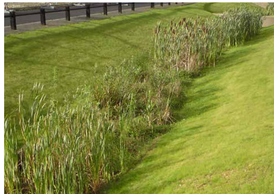
Example of a Swale
