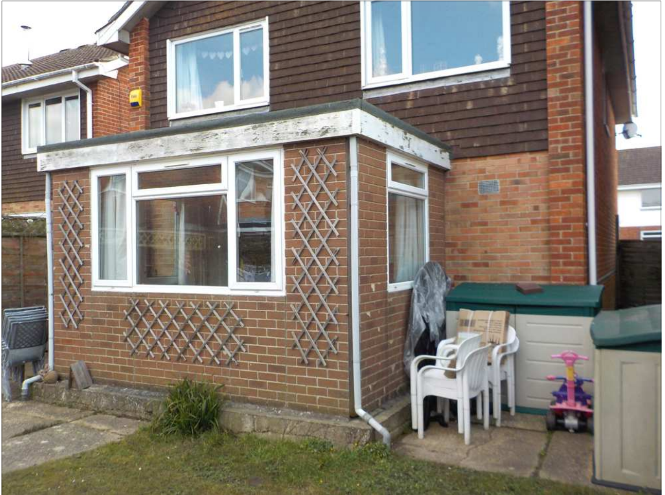
Rear of No. 49 Brook Gardens - shows existing rear extension
