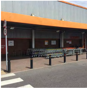
Sign 6 Signage Entrance Letters To left hand side of entrance
