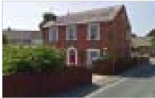
Red Brick Slate Grey Roofing with Window Surround and detailing
