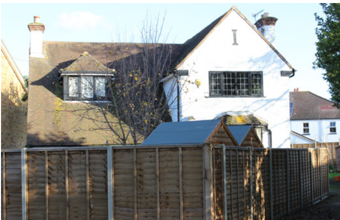
Photo 1: No. 48 Station Road (rear elevation)
