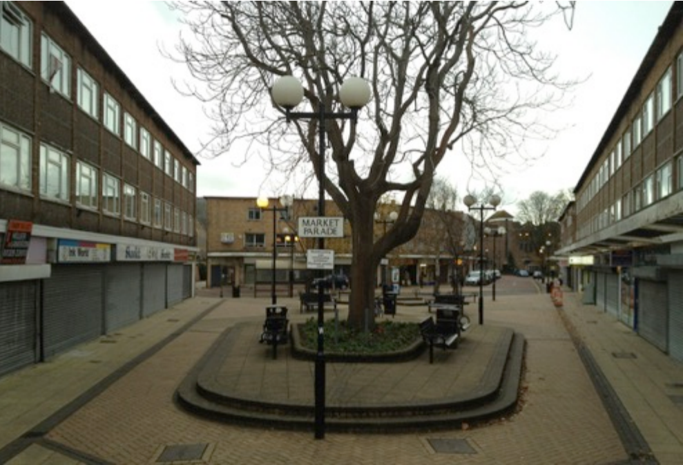
1. Existing Central Plaza viewed toward the Town Centre
