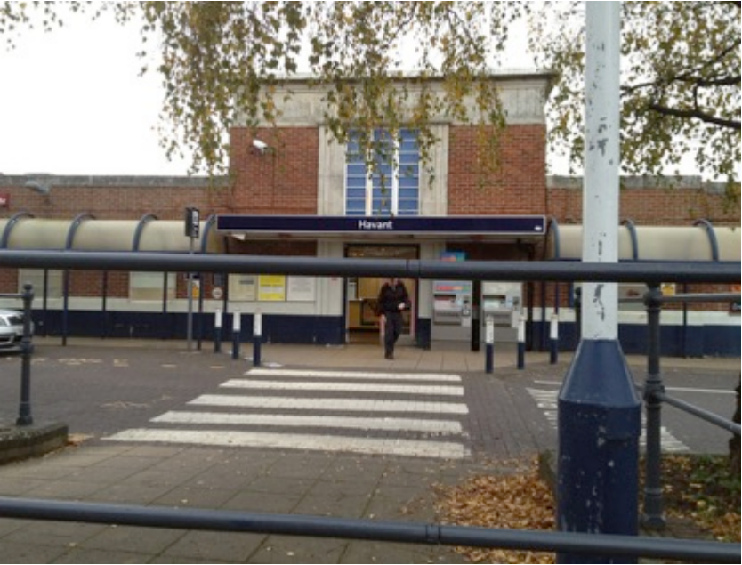
8. Existing Railway Station
