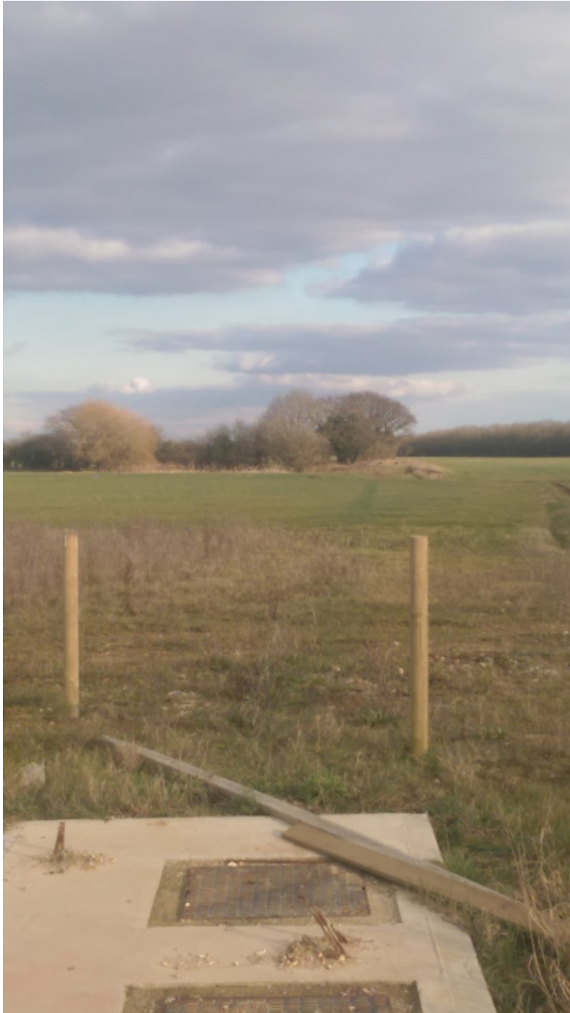
Image No.5 – Control structure and route of outfall to existing pond
