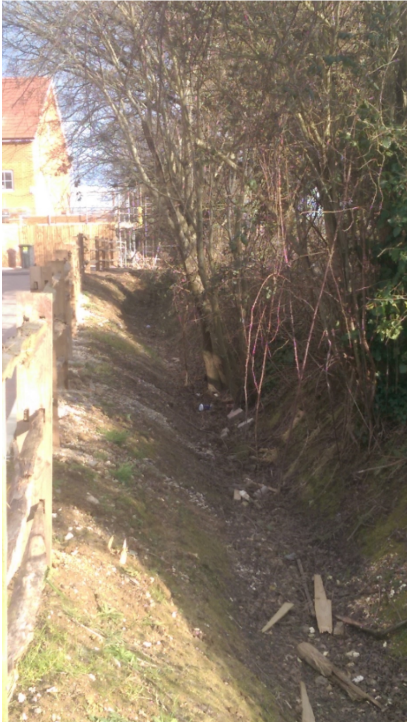
Image No.8 – Ditch between Manor Farm and Copsey Nursery cleaned out
