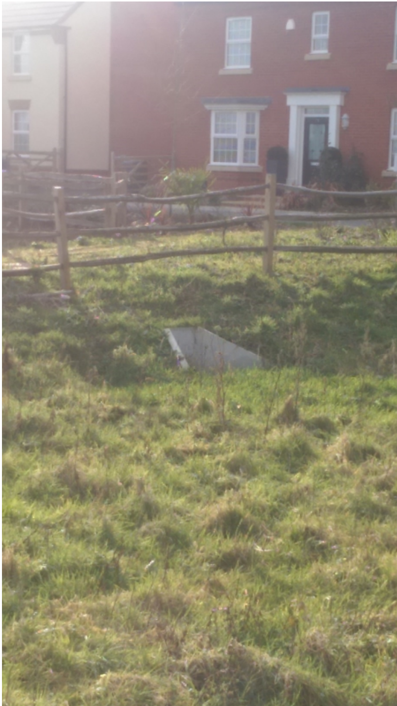
Image No.4 – Headwall link between ponds with protection fencing
