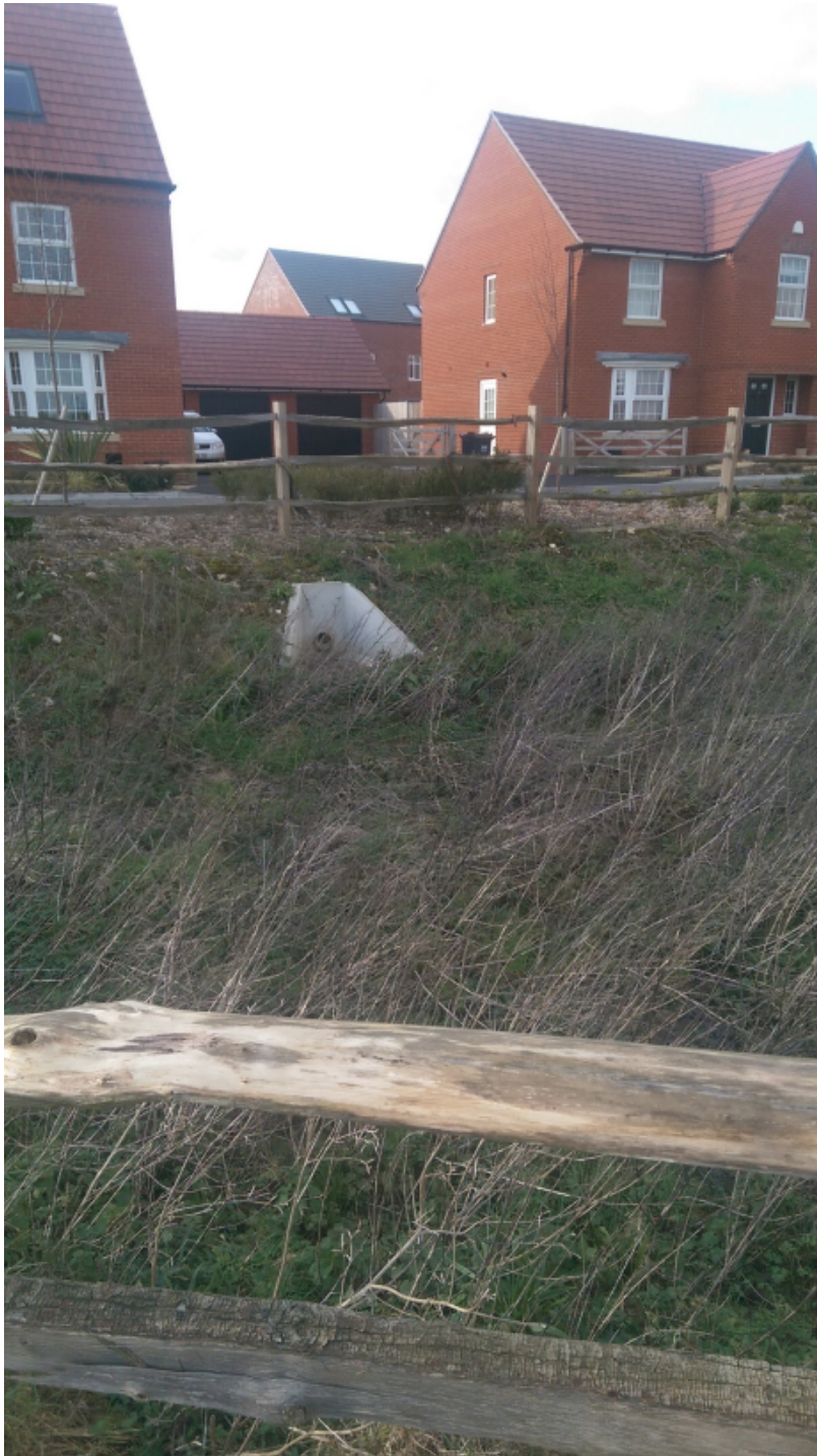
Image No.1 – Overflow from permeable carriageway with protection fencing
