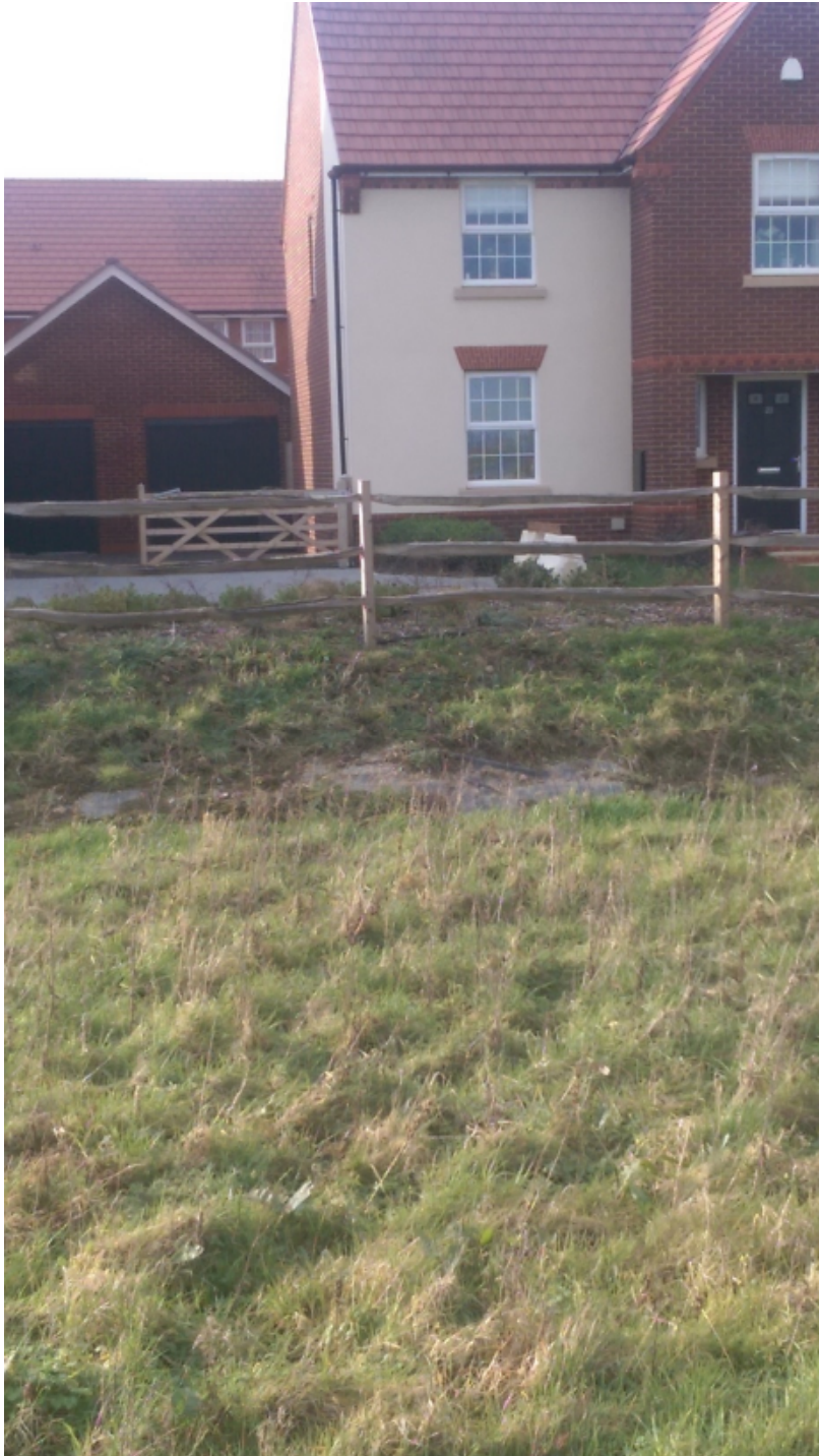
Image No.3 – Pond liner evident on embankment
