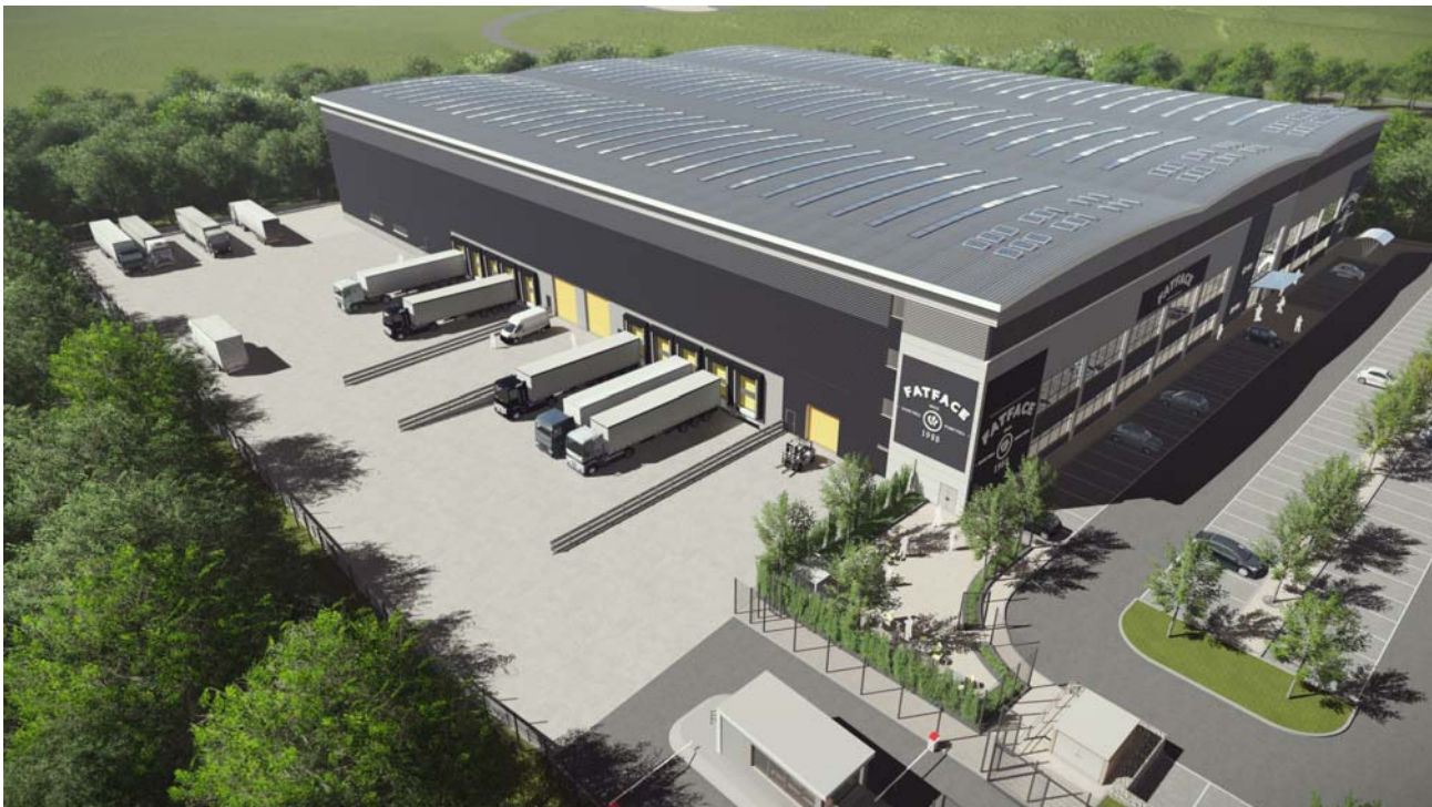
External Cladding Materials to Office and Service Yard Elevation
