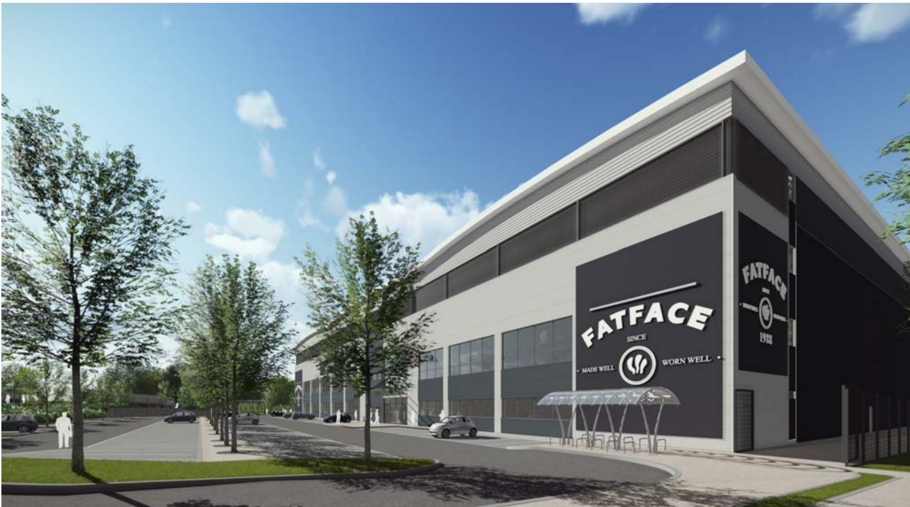
External Cladding Materials to Office and West Elevation
