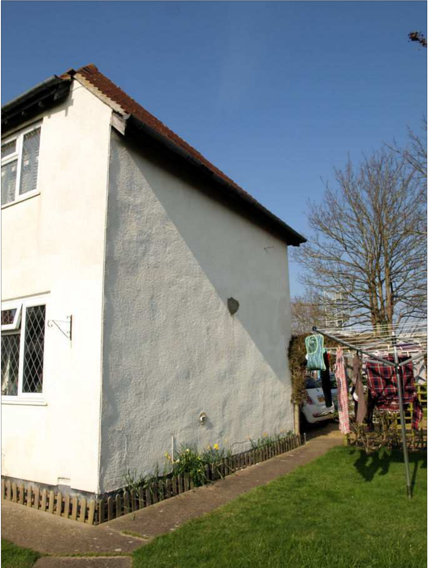
The side of No. 42 Park Way where the extension would go
