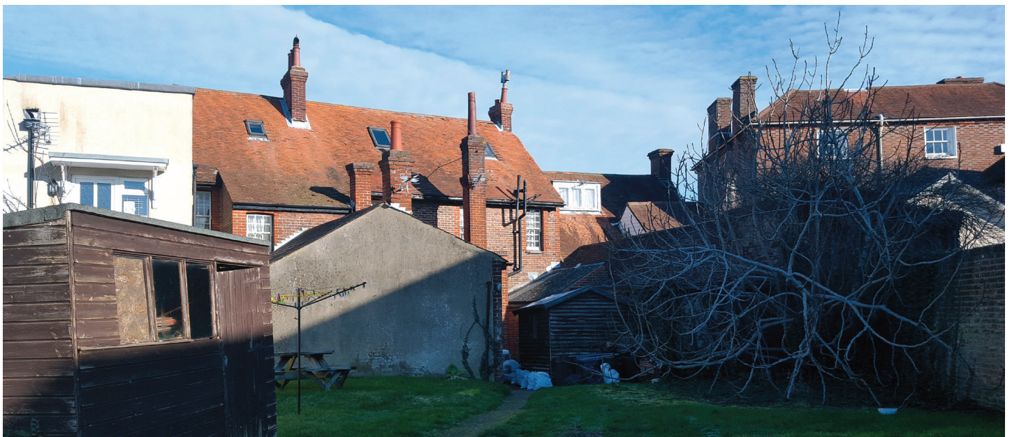
Rear elevation of Town Brewery
