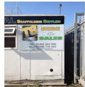
Mobile cabin (Offices)
