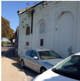
A1 Recovery workshop view from the street
