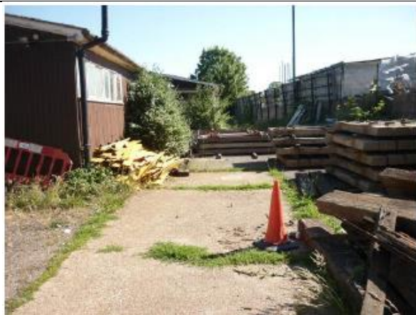
Photo 2: Derelict building and yard to the north East boundary of the site
