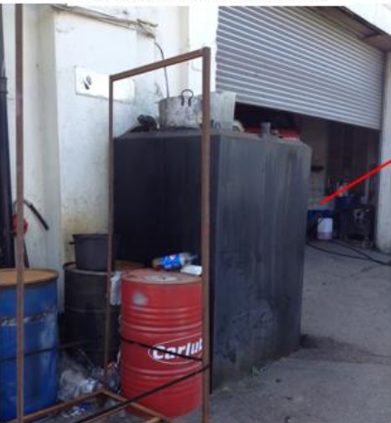
Above ground oil tank to the North east corner of the workshop
