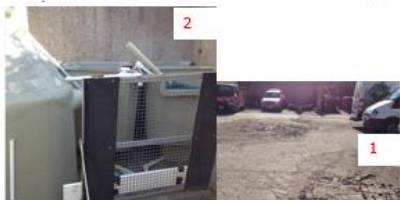
Former tank backfilled with concrete surfacing
