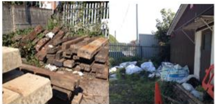
Derelict land and building structure with building material to the North East Boundary Of the site
