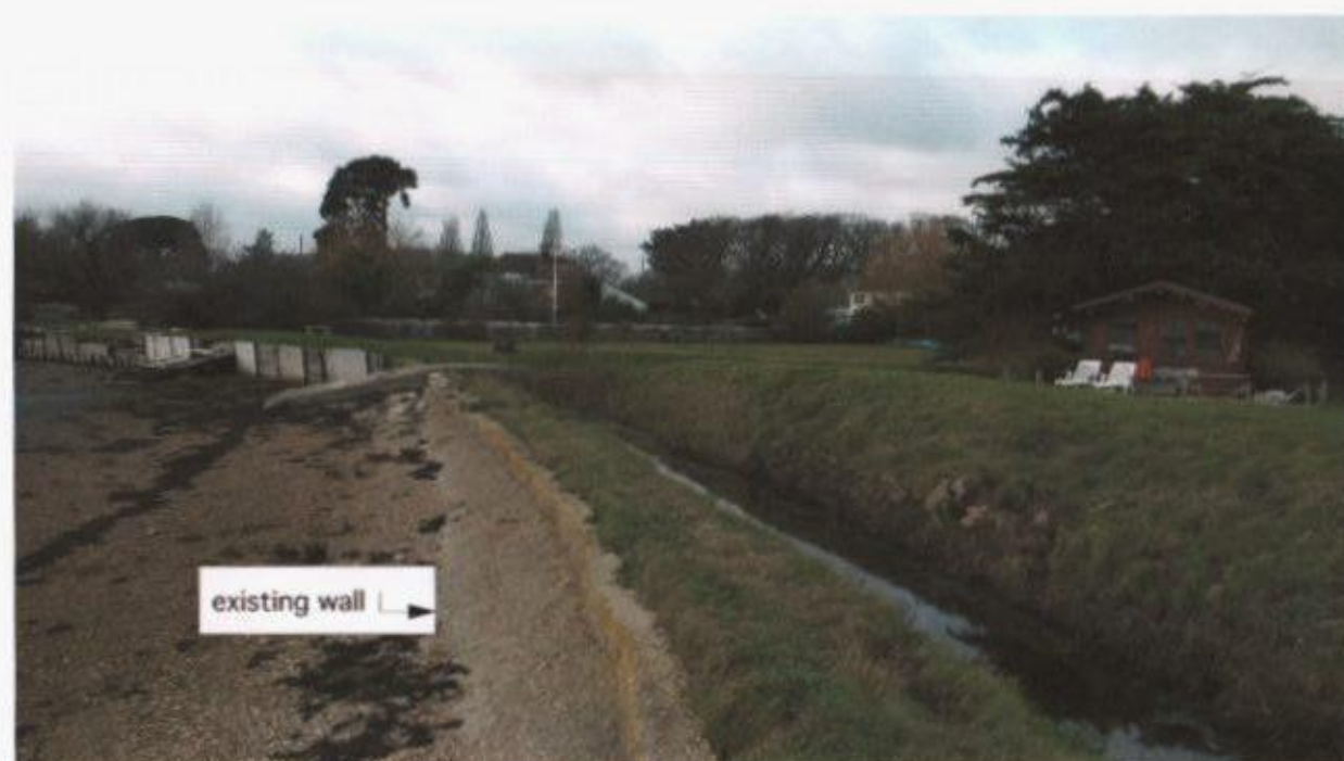
VIEW OF EXISTING - looking towards the WEST and showing ex ditch and wall.
