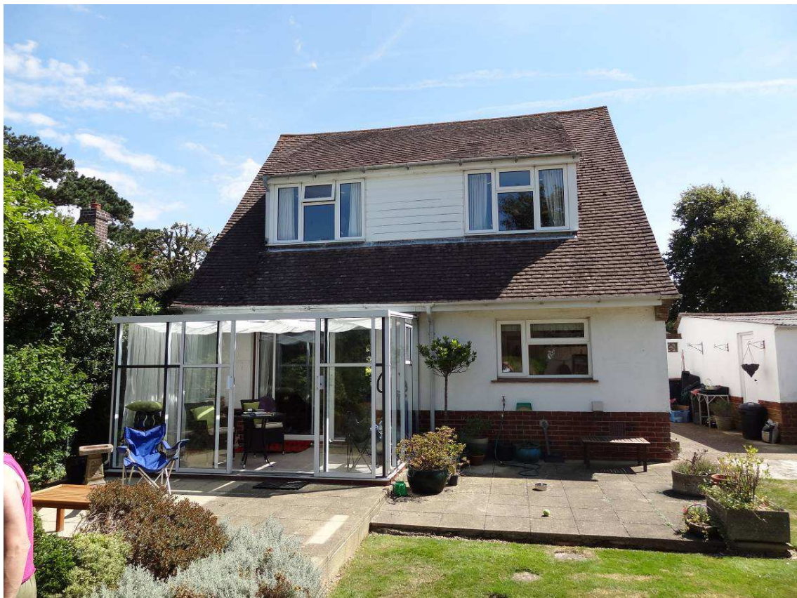
Photo 4 – View from rear garden of west elevation. Conservatory left of centre.
