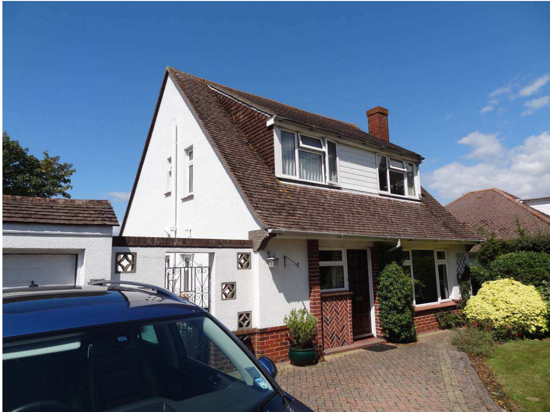
Photo 1 –View of the east elevation looking north-west. Adjoining bungalow to the north seen beyond.
