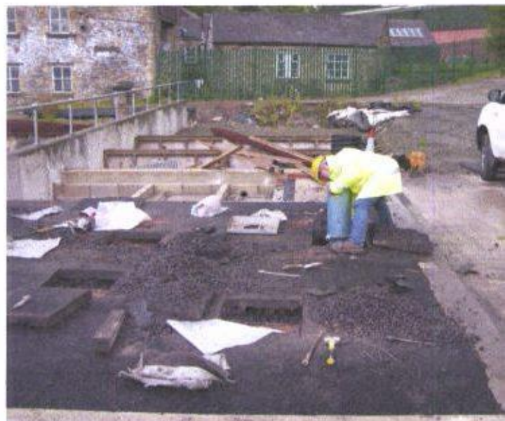
Figure 3 - In situ density tests post-trafficking
