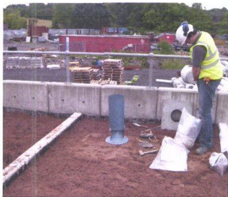
Figure 1 - in situ density test prior to construction of pavement
