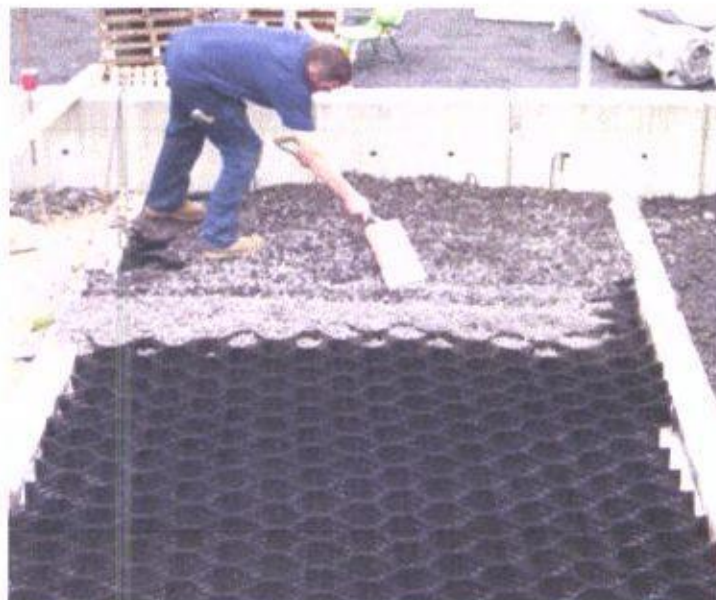
Figure 2 - Cellweb TRP® in construction
