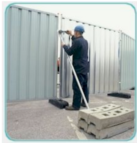
Figure 1: Galvanised metal hoarding
